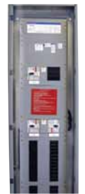
Wall-mount maintenance bypass panel
